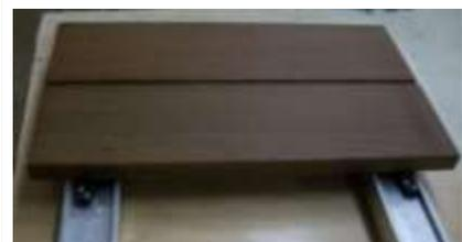
*After attaching the Deck Gliders to the deck boards, each deck board is then fastened to the Aluminum System Profile track, locking it in place.*
